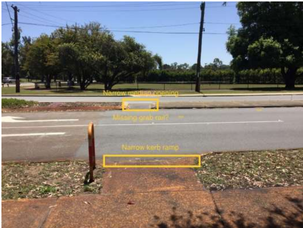
Above: Hamer Pde, east of intersection.
